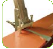
Stanchion installation complete
