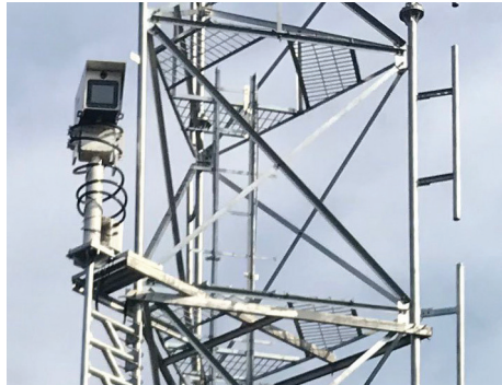
Hardware monitoring devices installed.
